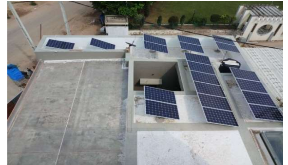
Residential Solar Rooftop Projects
